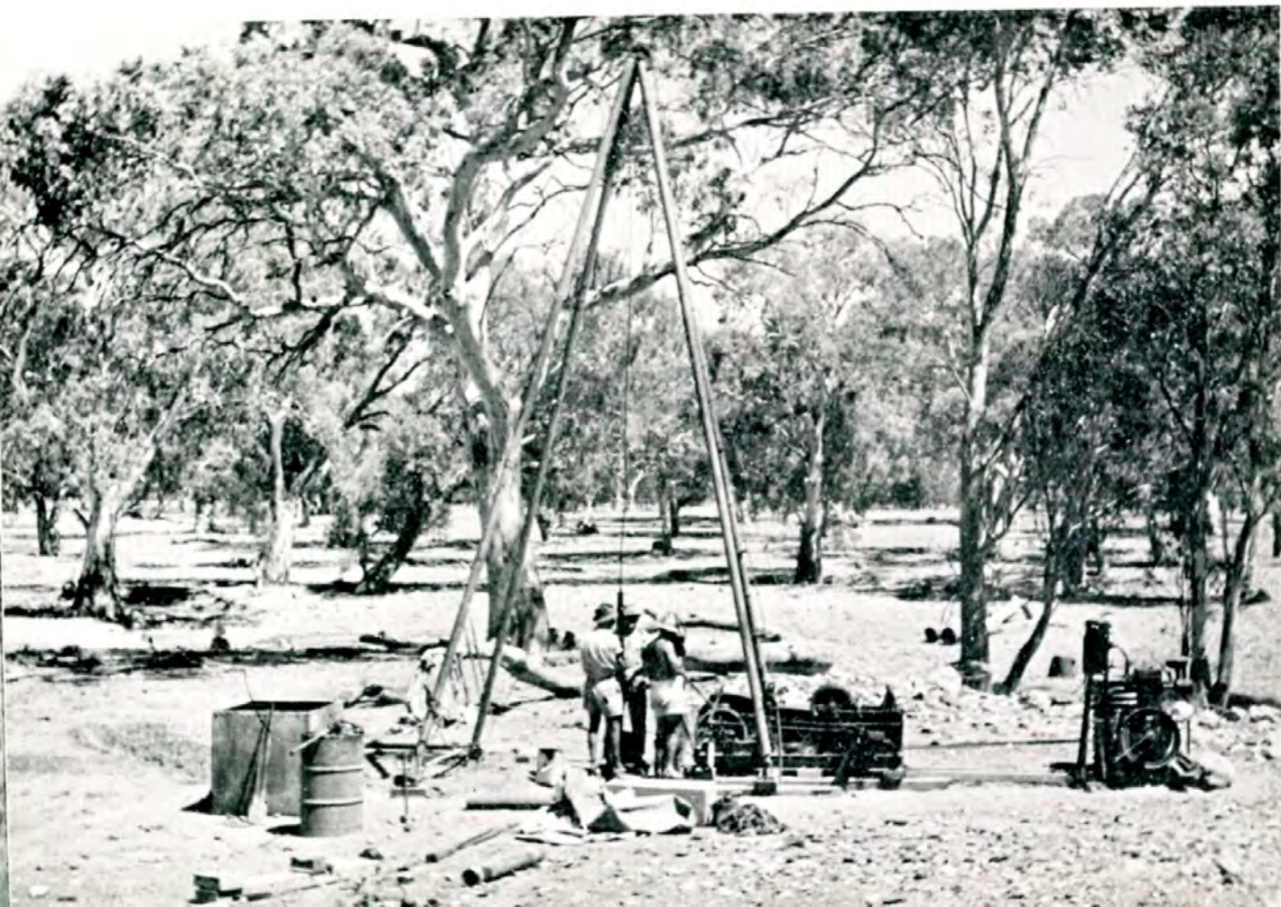
Plate 19.—Sinking Bore—Sliding Rock.
