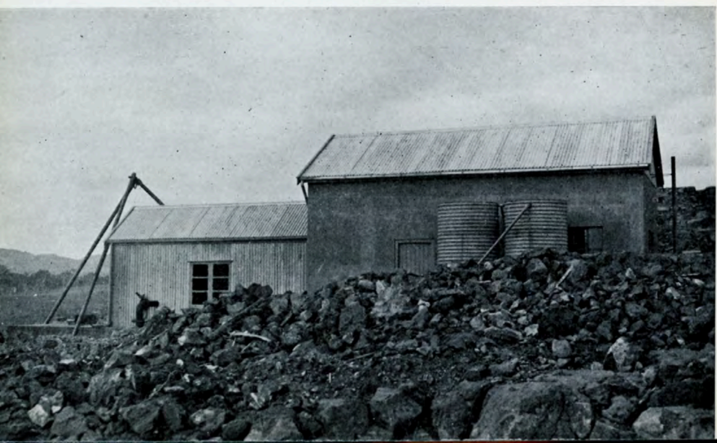
Plate 50.—Pumping Station, No. 2 Bore, Sliding Rock.
