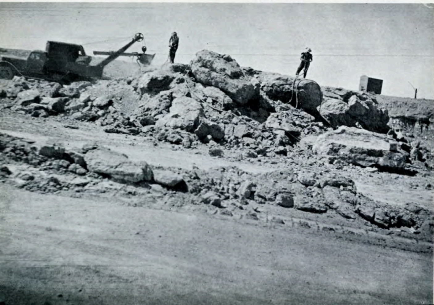
Plate 42.—Conglomerate Overburden—Open Cut.
