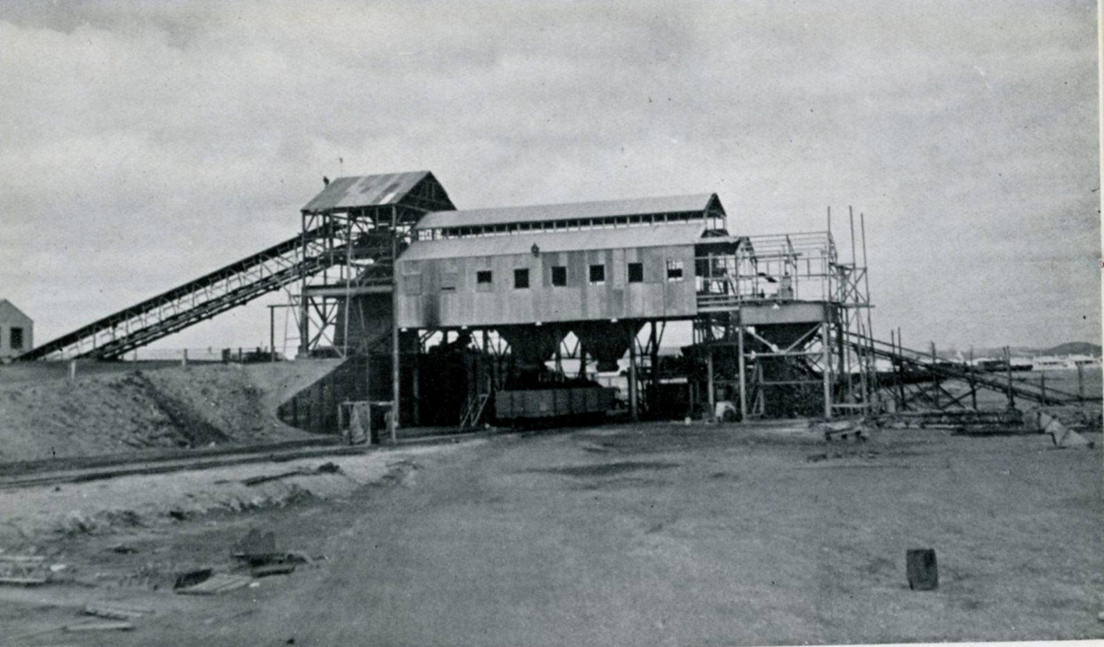
Coal Crushing and Screening Plant, Telford.
