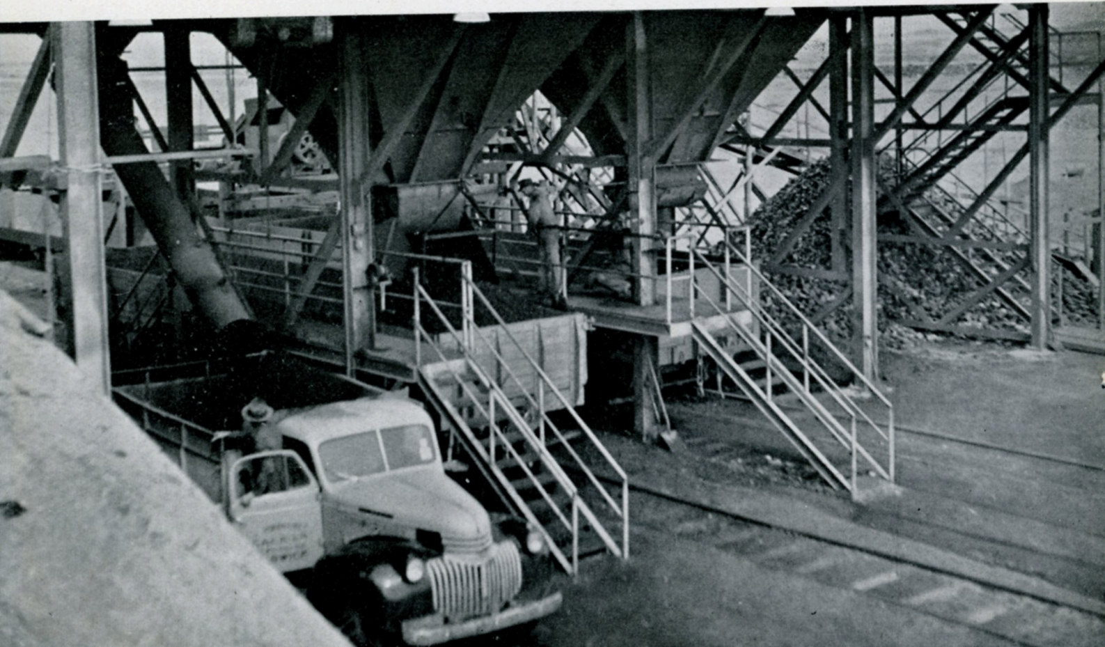
Loading Coal to Railway Trucks.
