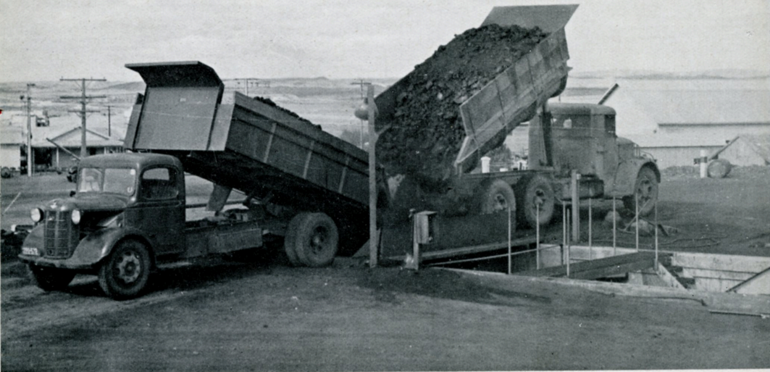
Tipping Coal at Crushing and Screening Plant.
