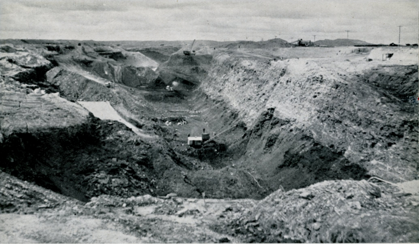
Telford Open Cut.
