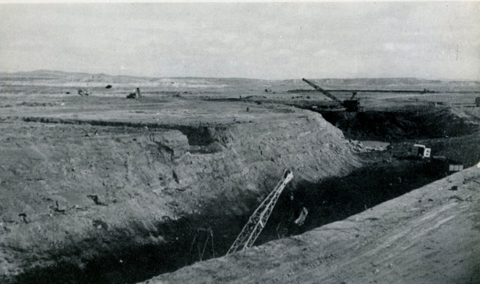
North Field Open Cut.
