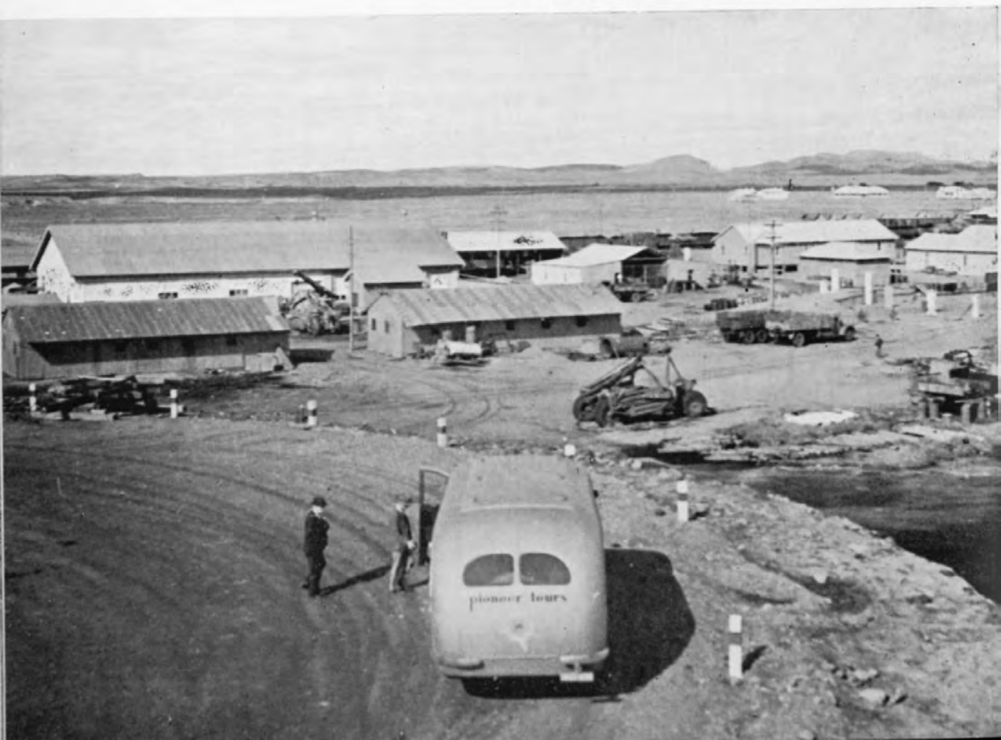
Workshop Area from Crushing and Grading Plant.
