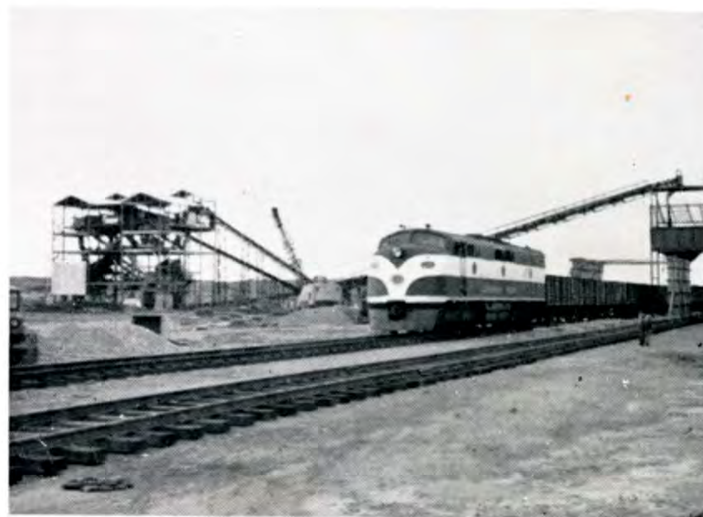
Coal train at new grading plant.
